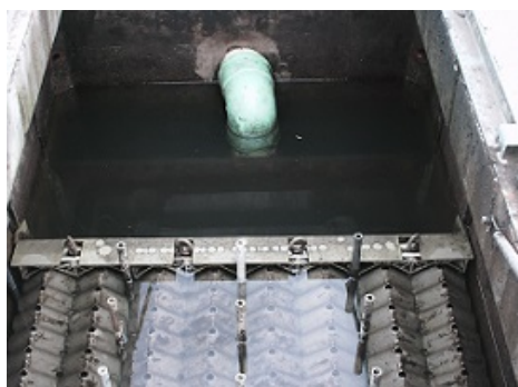
Figure 1. Oil-water separator (Stormwater Partners SW Washington)
