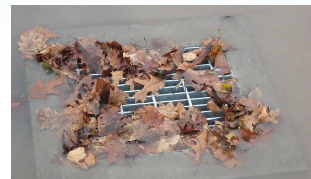
Leaf Debris Covering Overflow
