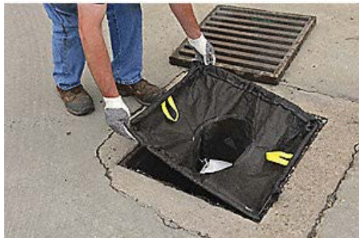
Figure 1. Drain inlet insert (Grainger)
