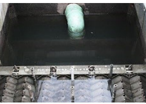
Oil water separator (Stormwater Partners SW Washington)
