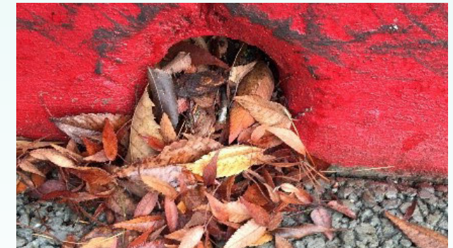
Leaves Clogging Inlet Pipe
