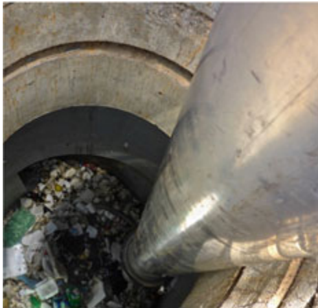
Figure 1. Hydrodynamic separator (EPA)
