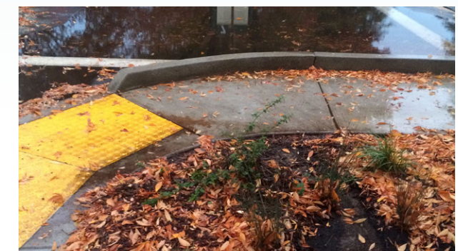
Sand and Sediment Entering SCM Drainage Area
