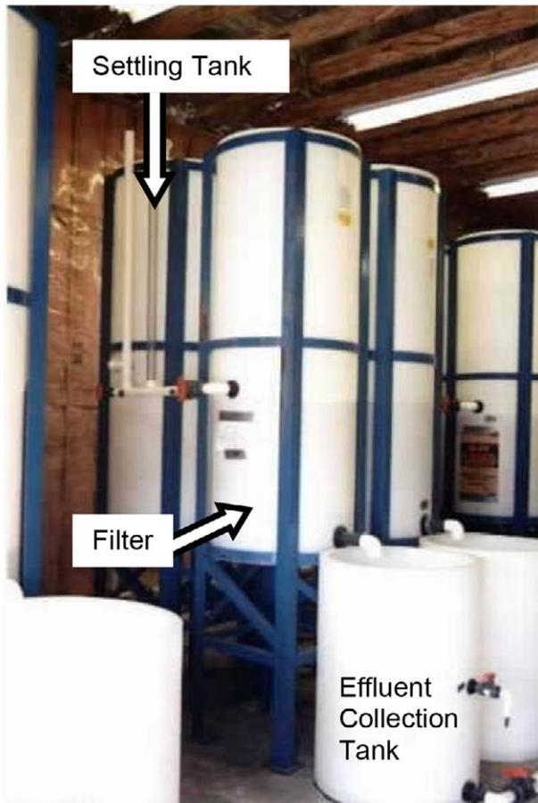
**Figure 4. Typical non-mechanized treatment unit.**
