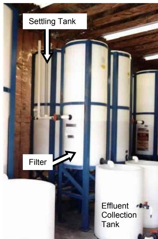
Figure 4. Typical non-mechanized treatment unit.
