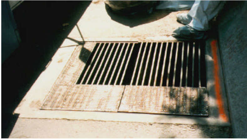
FIGURE 2 Modified drain inlet.
