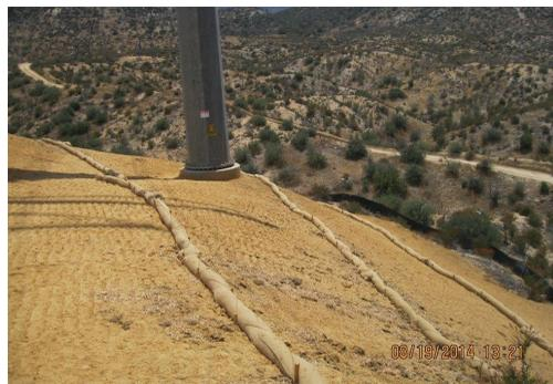
**Figure 8: Application of hydromulch at 5,000 lb/acre, with burlap wrapped fiber rolls installed using the Caltrans Type 2 method**
