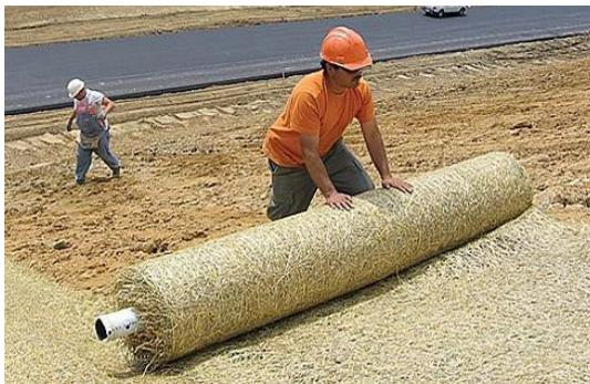
**Figure 7: Rolled erosion control product installation**
