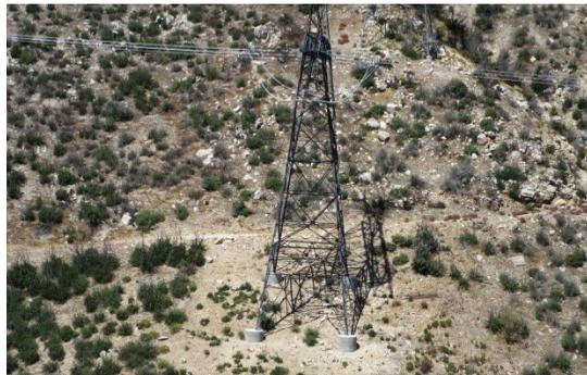
**Figure 12: Project site that meets the final stabilization condition. Demonstrated using RUSLE2 with rocky terrain and partial vegetation as justification.**
