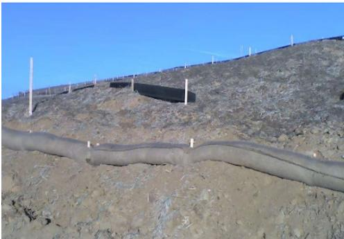
**Figure 11: Project site that demonstrates failed hydromulch application. This site does not qualify for final stabilization.**
