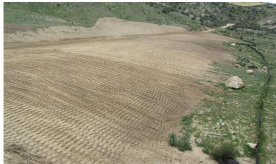
**Figure 5: Decompacted and track walked slope is well prepared for hydroseed application**
