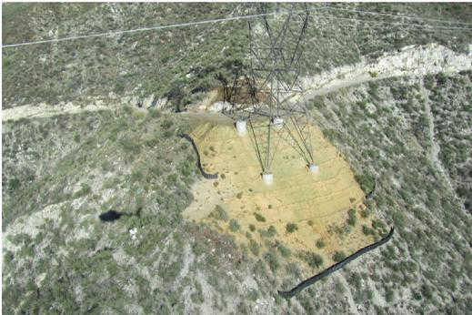
**Figure 13: Steep slope that meets the final stabilization condition. Demonstrated using RUSLE2 with hydromulch, fiber rolls, and perimeter controls as justification.**
