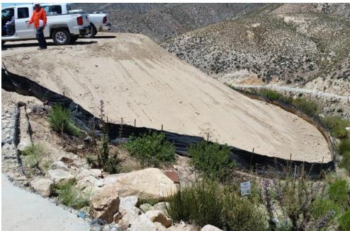
**Figure 4: Perfectly smooth slope is not an ideal surface for hydroseeding**
