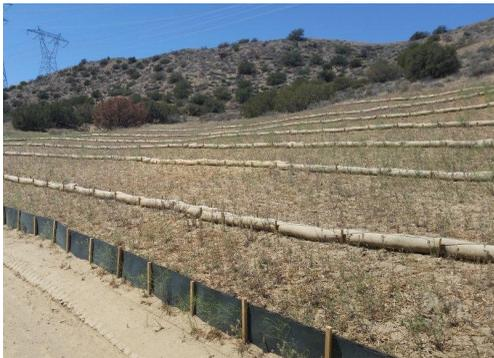
**Figure 1: Slope recently hydroseeded with native seeds**
