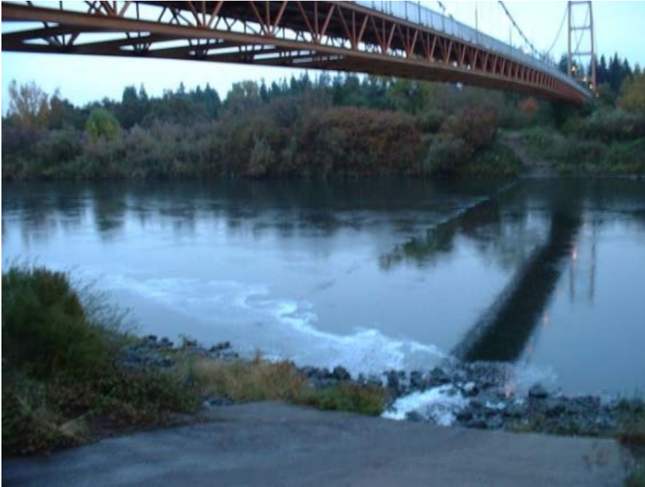
Outfall – Guy West Bridge
