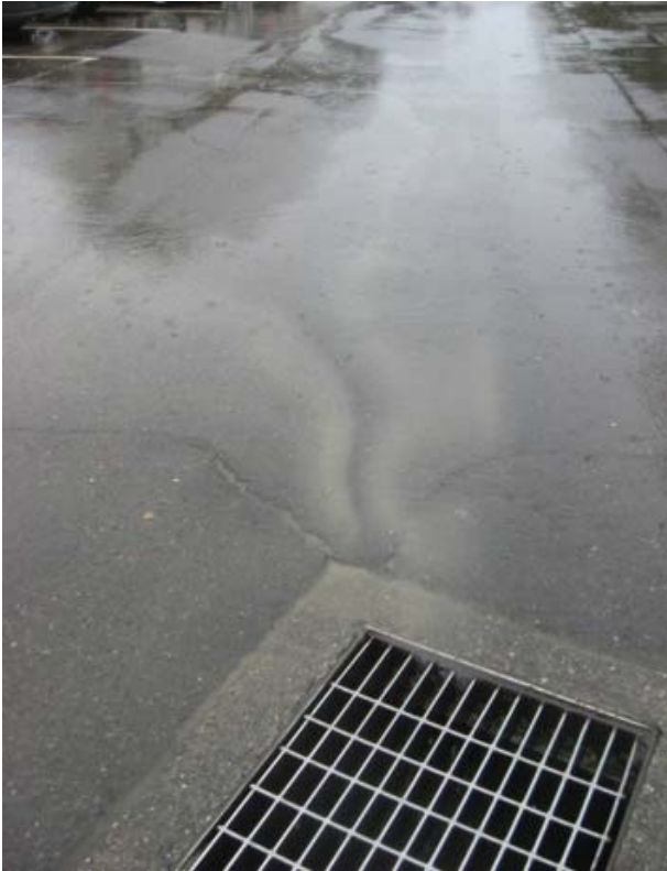
Drain Inlet - Campus
