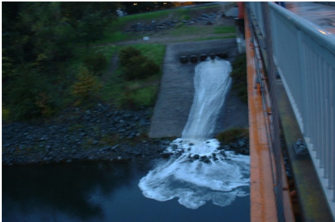
Storm Drain Discharges into American River
