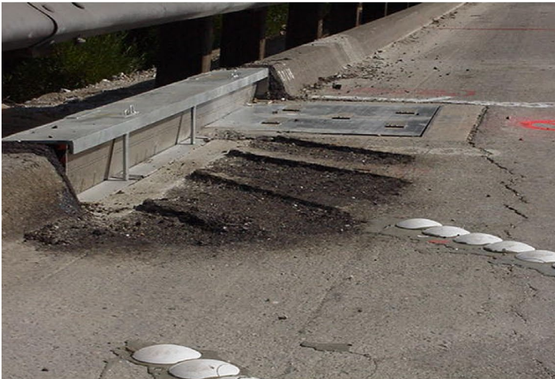
Figure 2 Litter Inlet Deflector
